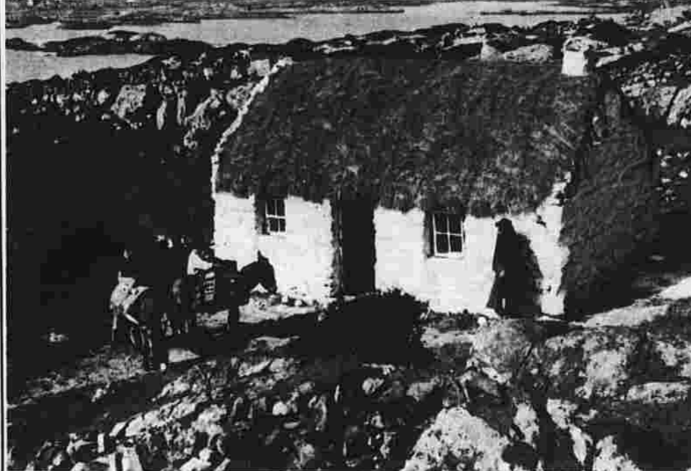
A thatched cottage in Connemara in the West of Ireland. The cottage is typical of the region — thatched and whitewashed. The type of thatching varies according to the region, and is often carefully pegged down to resist the winter storms.
